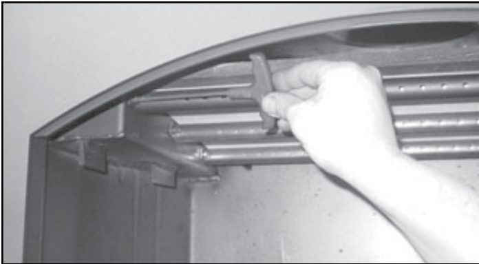
Figure 31.2 Removing Manifold Tube
